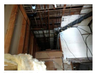
**Photo #17** View of first floor water damaged ceilings (building 211).
